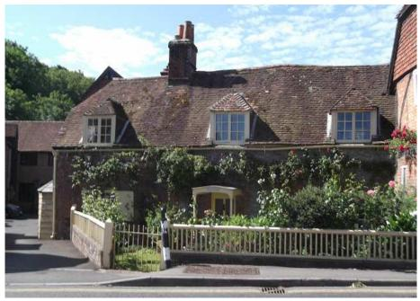
It has a tile roof, half-hipped at the east end and a catslide at the rear, and hipped dormers. The north front elevation is of one storey and there is an attic with three casement windows. The doorway, (replacing a former window), has a half-glazed door within an open porch, having a canopy on slender cast-iron columns. At the east end there is a single-storied extension, with boarded walls and hipped slate roof. Inside, the frame is partly exposed.
