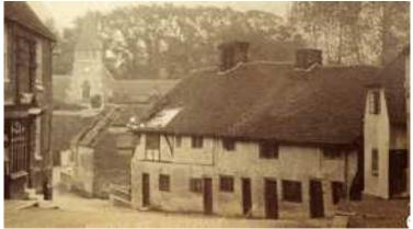
The most complete example of a Wealden House in the local area. A jettied three bay house with single bay hall forms Nos.10 and 11, No.9 being a latter extension. They are timber framed with plaster infill and with later brickwork cladding. Timbers have been dated by dendrochronology to c1495.
